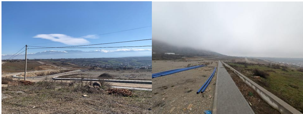
Figure 1 Field photo - Rahovec Industrial Park (Opterushë)
